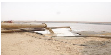
Figure 16: Waste pit (Drilling Y, 2017)
