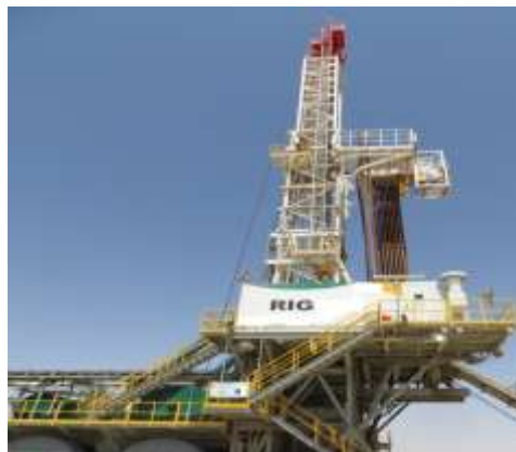
Figure 3: On-Shore Drilling rig, (Company X, 2017)
